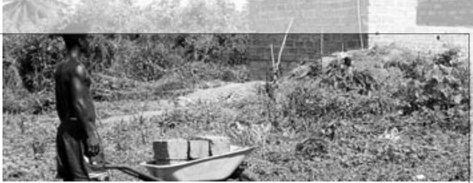
UNHCR is helping former IDPs to rebuild a school in Balama, Liberia. UNHCR/A. Rehr
