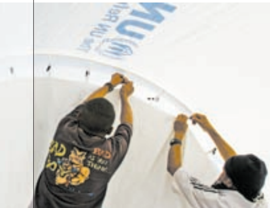
UNHCR's ERTeam quickly set about improving shelter in some of Dili's most congested makeshift encampments. Photo: UNHCR/N. Ng
